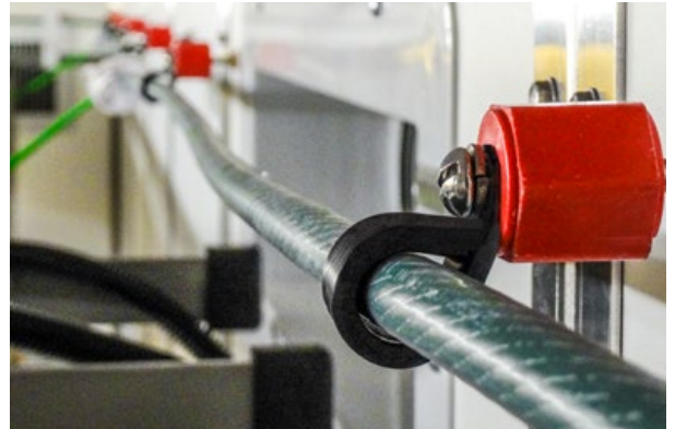
Halo Ground System for AP FORT® Shelter Series
